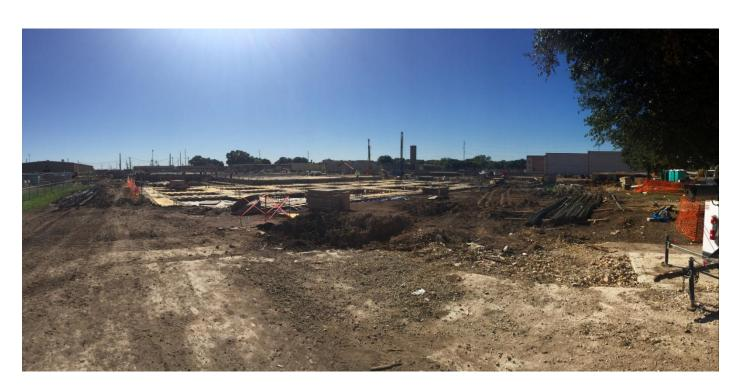
**FOUNDATION** – Moisture protection and under-floor mud slab concrete installations continue. Formwork is being installed at the New Weight Room and Large Group Instruction (LGI) Room.
