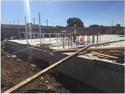
PLUMBING – The Secondary Gym foundation was poured 2 weeks ago. Plumbing rough-in installation is in progress.
